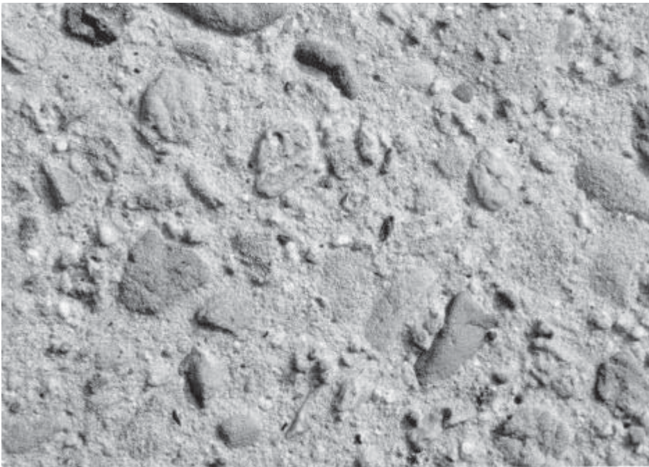
Figure 3-2. Textured finish by sandblasting
