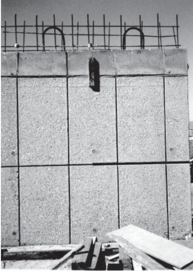
Figure 2-2. Example of field mockup sample
