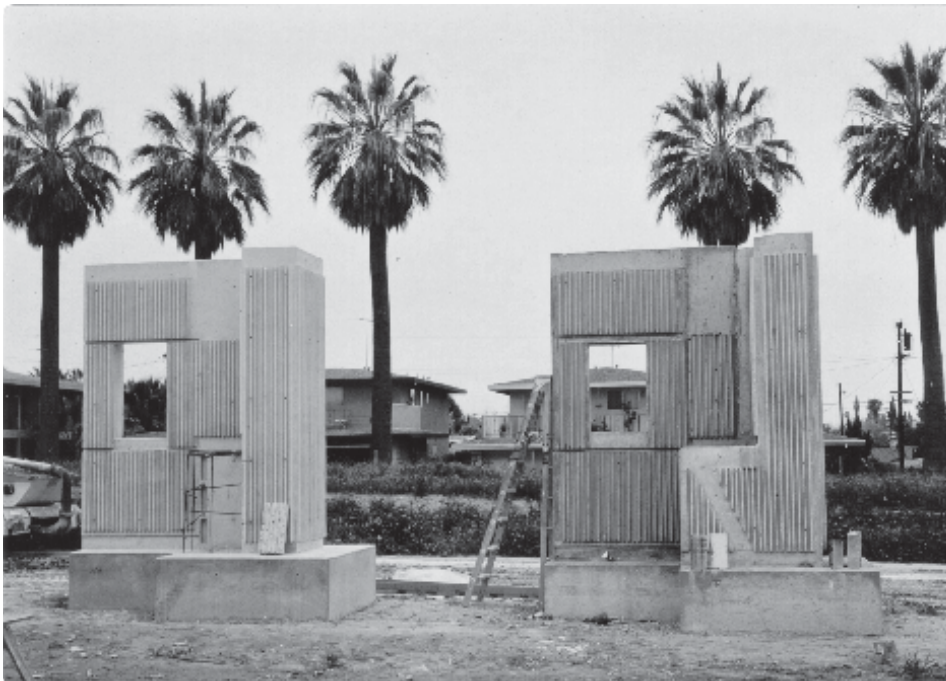
Figure 5-1. Illustration of contamination of light architectural cement with regular gray cement (uncontaminated field mockup on left)
