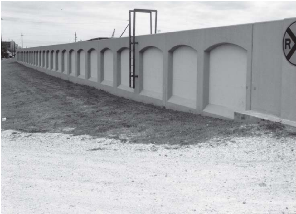
Figure 11-2. Painting of concrete highlights arches in floodwall
