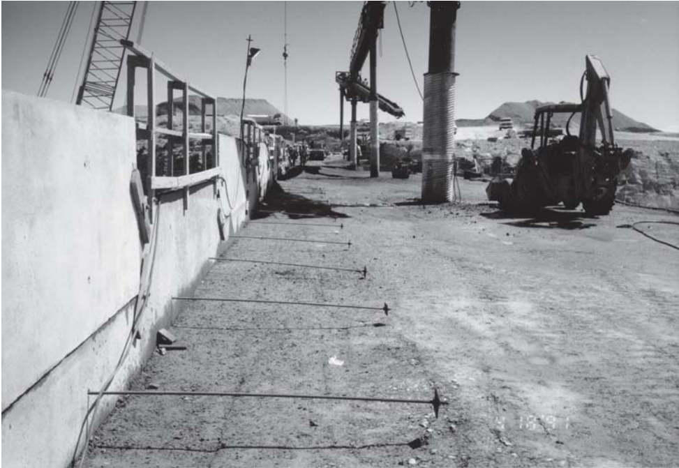
Figure 11-5. Form anchors in RCC placement
