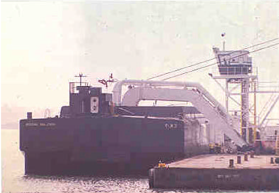
Figure 2. The Pump Barge Liberty Offloading a Sediment Scow at the Sonoma Baylands CDF Site in the Bay Area.
