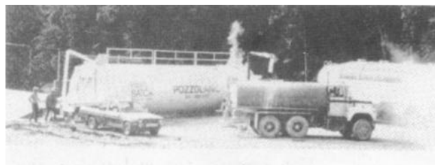
Figure 4-34. Portabatch lime slaker.
