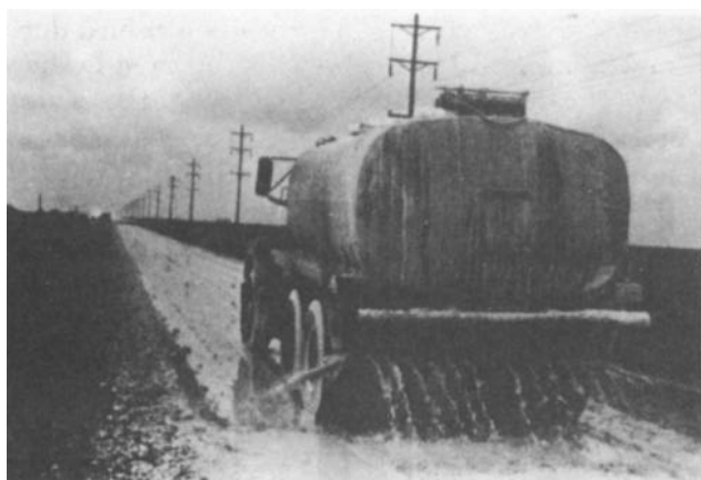
Figure 4-31. Spreading of lime slurry.
