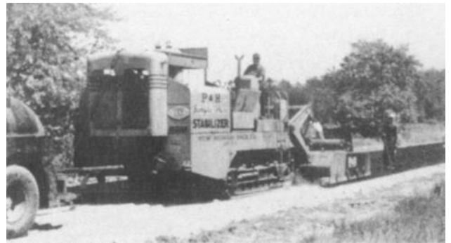
Figure 4-46. Multiple rotary mixer.
