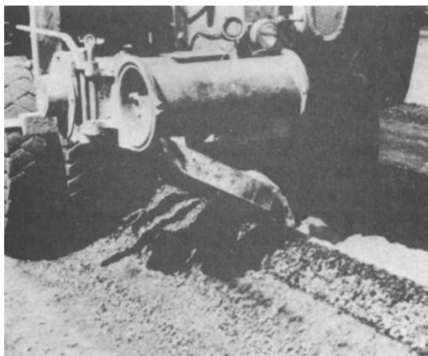
Figure 4-9. Windrow-type mechanical spreader placing cement on windrow.
