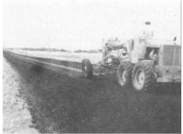
Figure 4-50. Mixing with motor grader.
