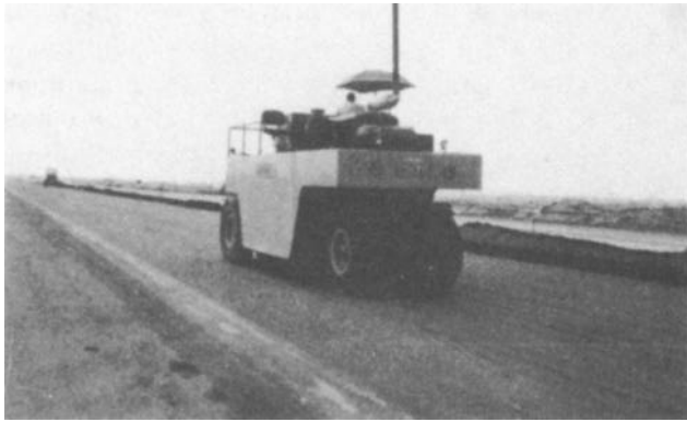
Figure 4-42. Pneumatic roller completes compaction of LCF base.
