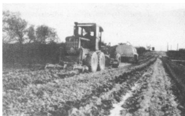
Figure 4-33. Grader-scarifier cutting slurry into stone base.
