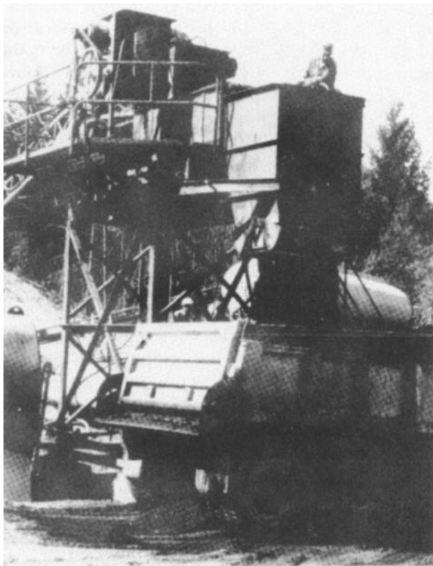
Figure 4-53. Stationary cold-mix plant.
