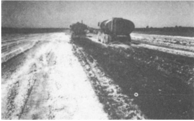
Figure 4-35. Watering of lime-treated clay on airport project.
