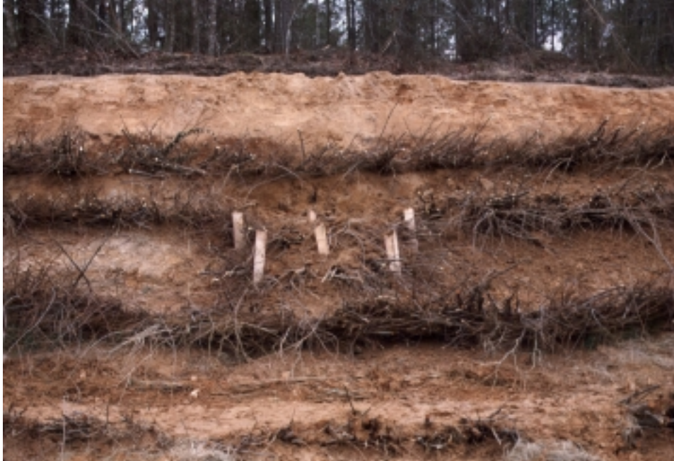
Figure 18-15a Newly installed system
