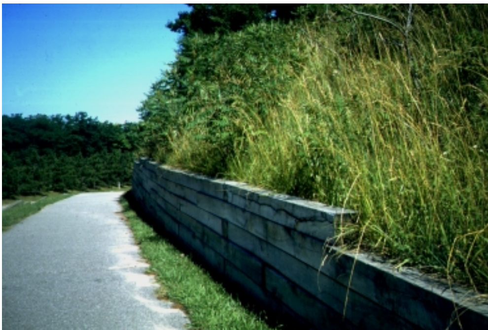
Figure 18-26 Low wall at the base of a slope with vegetation on face of slope (Donald H. Gray photo)
