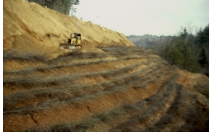
Figure 18-1b Measures being installed
