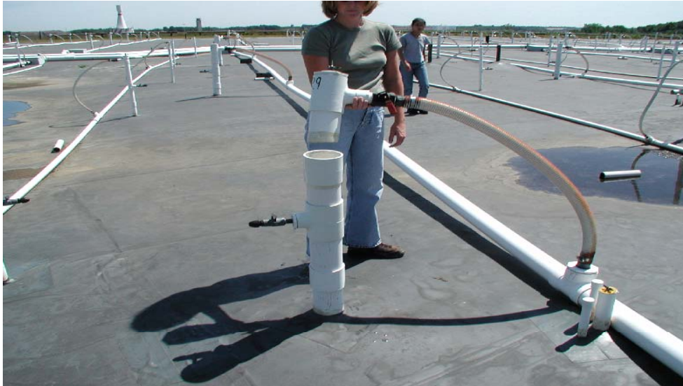
Soil Vapor Extraction System
