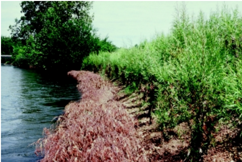
Figure 16-21b Tree revetment system with dormant posts, 2 years after installation
