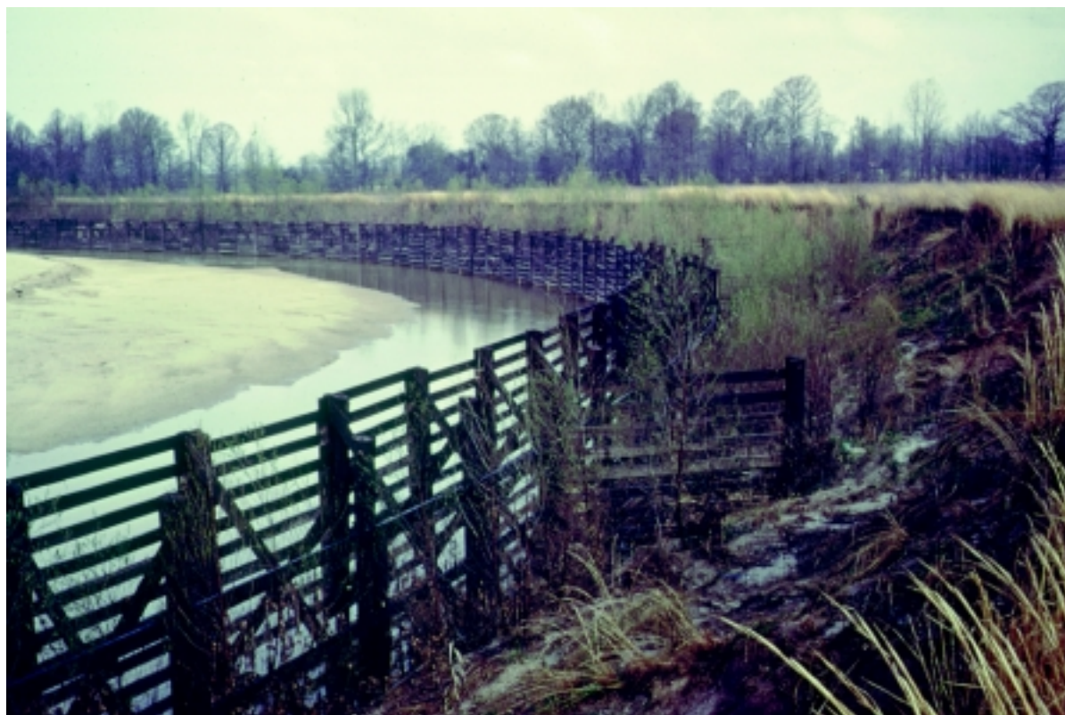
Figure 16-28 Slotted board fence system
