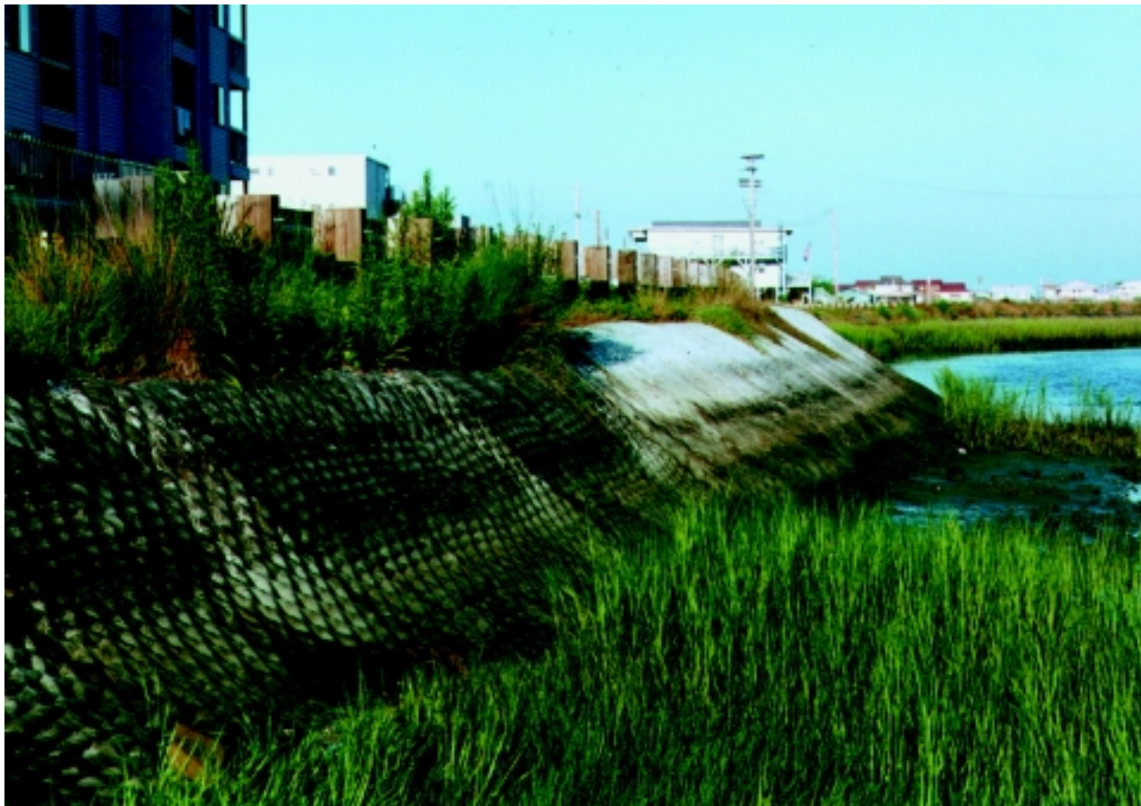
Figure 16-50 Concrete revetment (poured in place)
