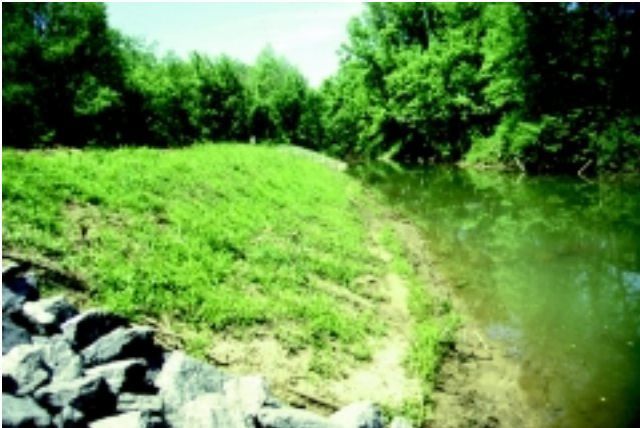
Figure 16-19c Brushmattress system 6 months after installation (Robbin B. Sotir & Associates photo)
