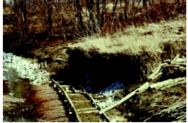
Figure 16-15b A live cribwall during installation
