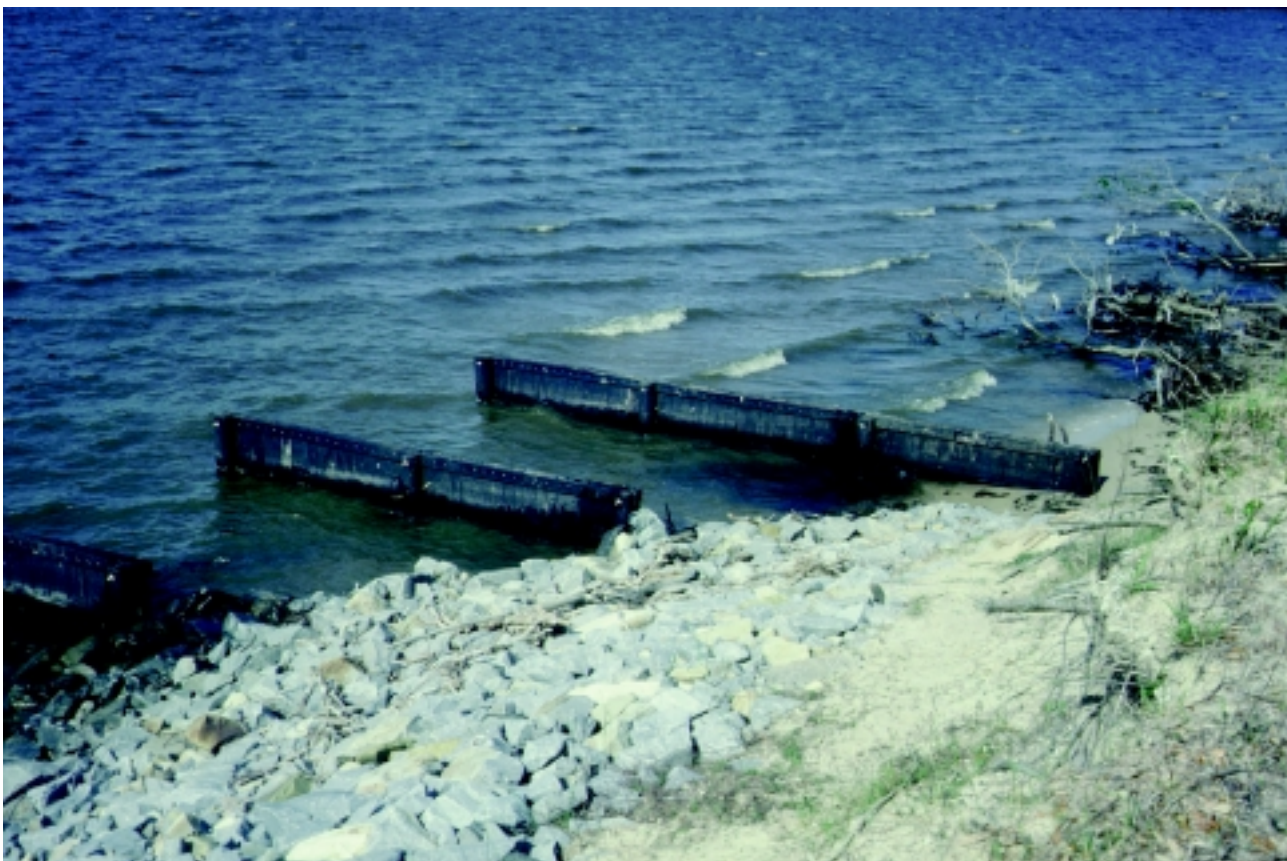
Figure 16-45 Timber groin system
