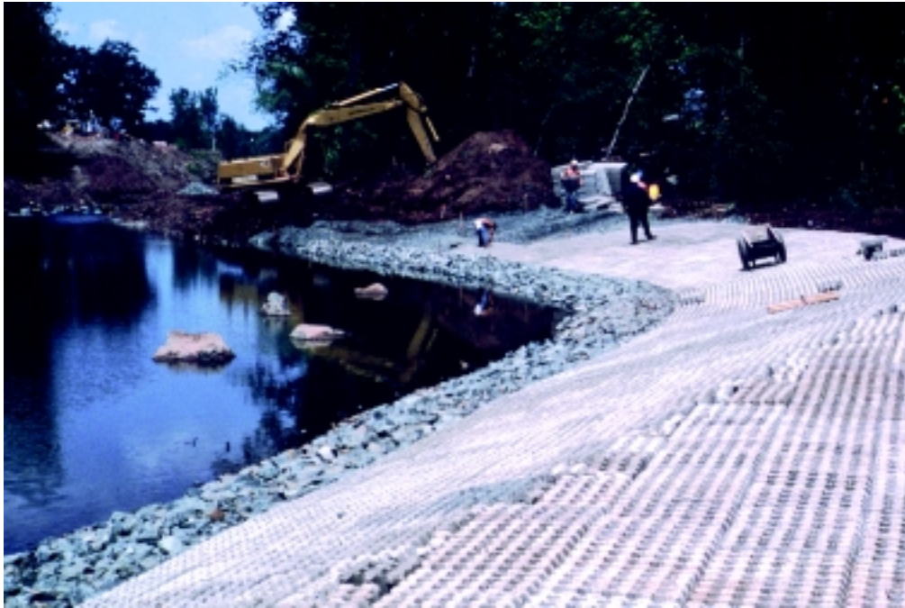
Figure 16-35a Concrete cellular block system before backfilling
