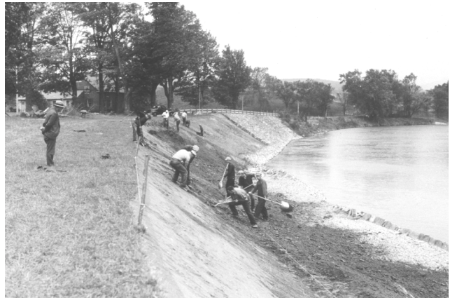
Figure 16-3b Bank shaping prior to installing soil bioengineering practices, Winooski River, Vermont, September 1938
