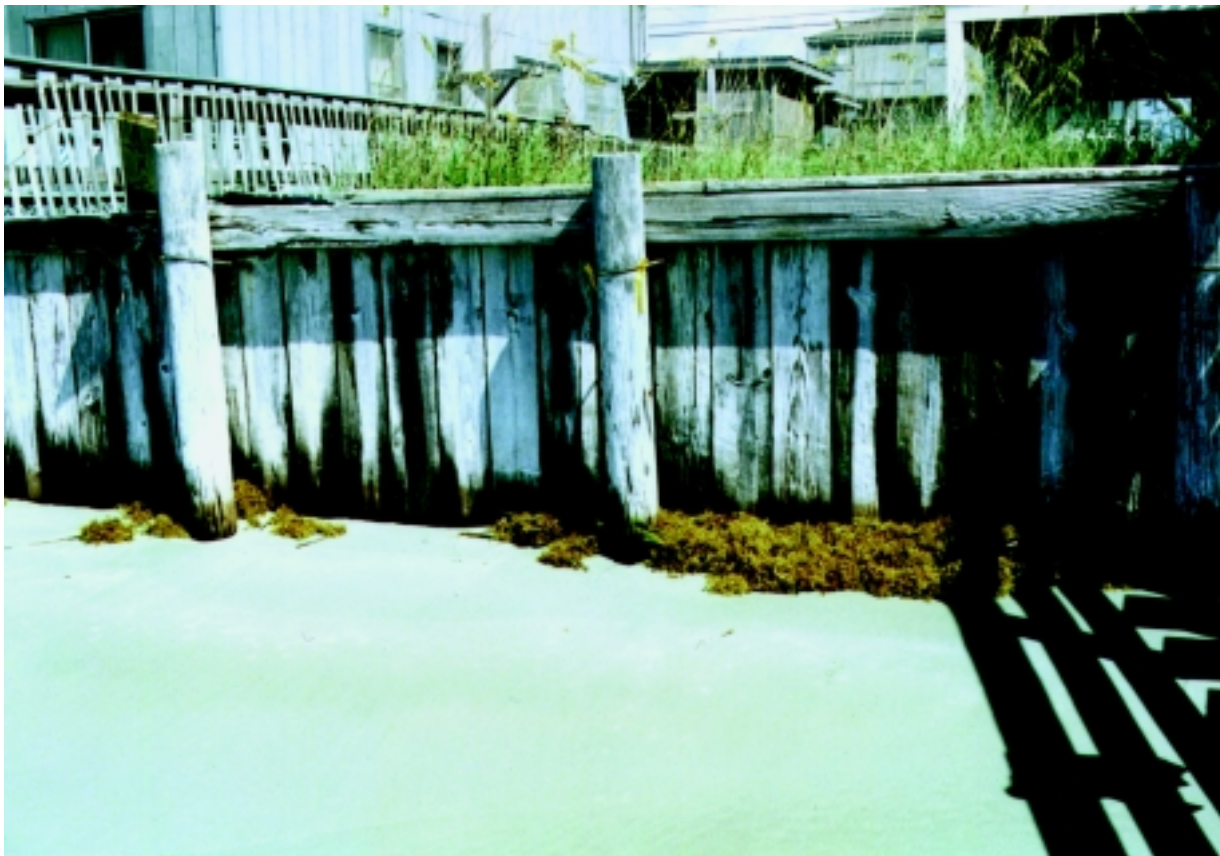
Figure 16-46 Timber bulkhead system
