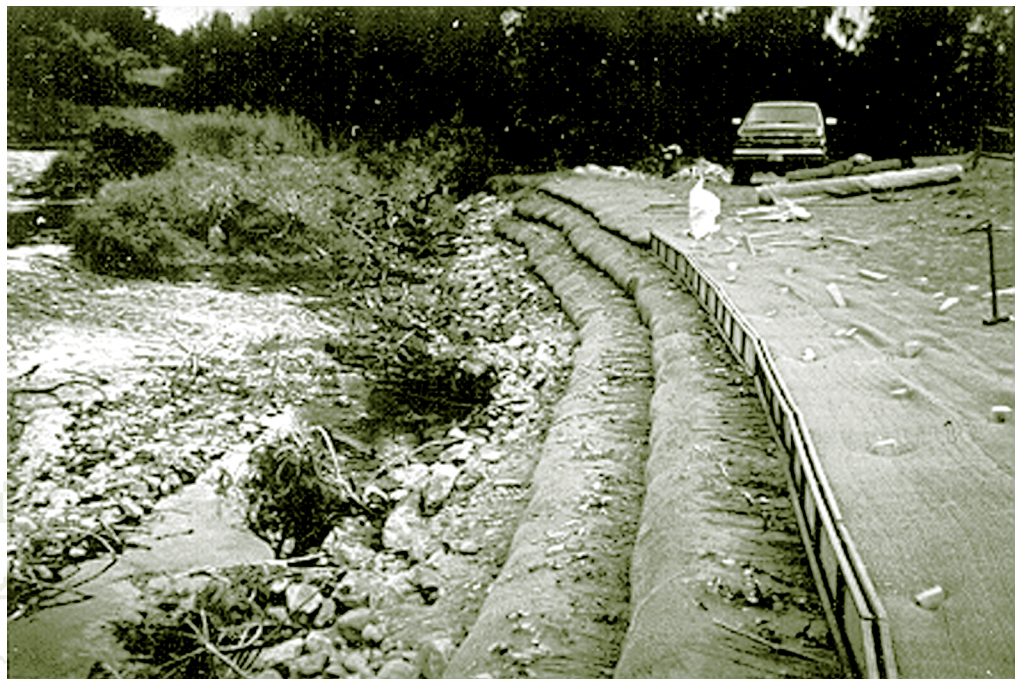
Figure L-1. Salmon Creek bank protection using rock toe, soil-reinforced lifts and vegetation.
