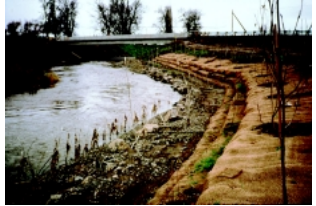
c. Soil Reinforcement lifts with rock toe. Touchet River. 2000.
