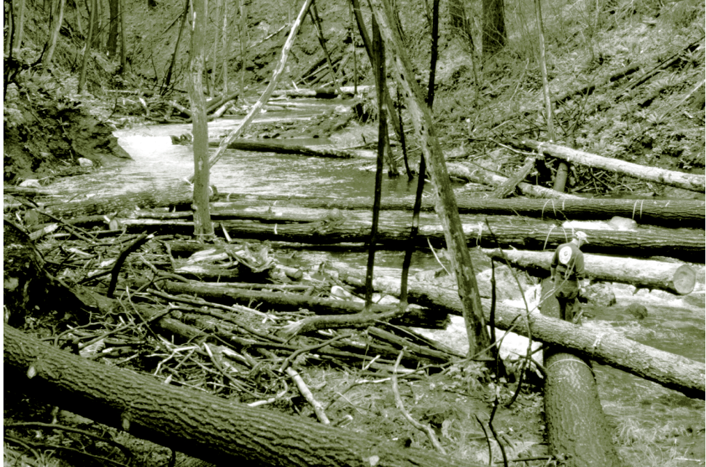
Figure L-2. Engineered log jams on Whatcom Creek.
