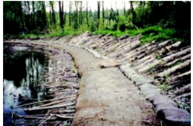
d. Soil Reinforcement lifts with woody plantings. Cedar River side channel.
