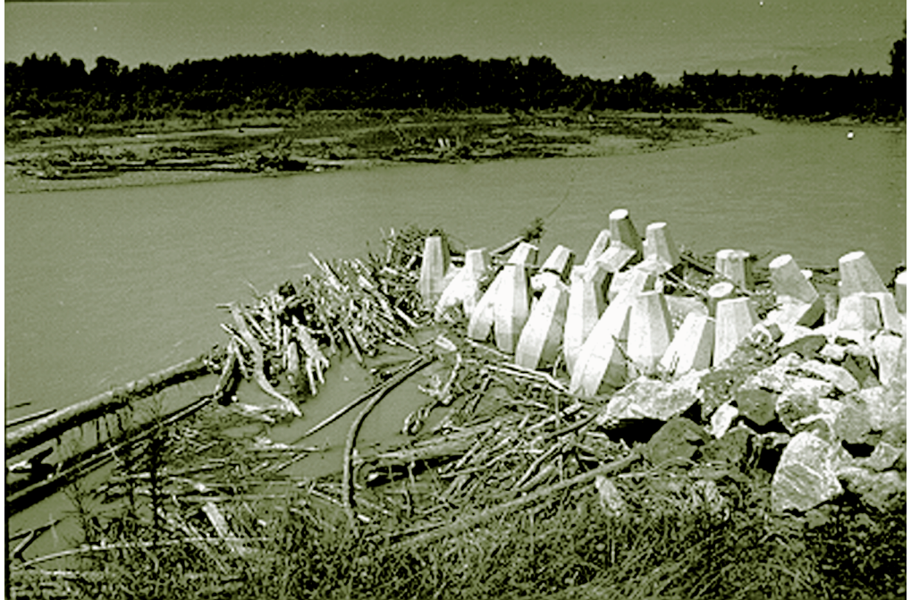
Figure L-3. Concrete dolo groins on the Nooksack River.
