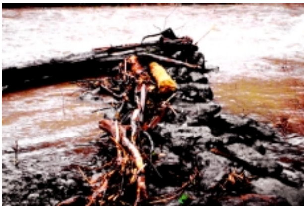
c. Rock Groin with woody debris accumulation. Big Quilcene River. 1998.
