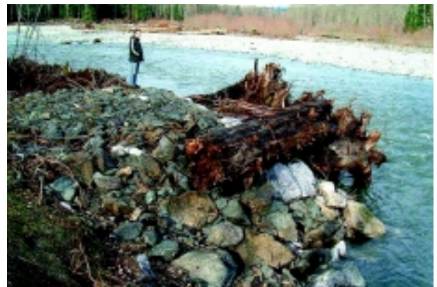
e. Large Woody Debris embedded in Groin. South Fork, Nooksack River. 2002.
