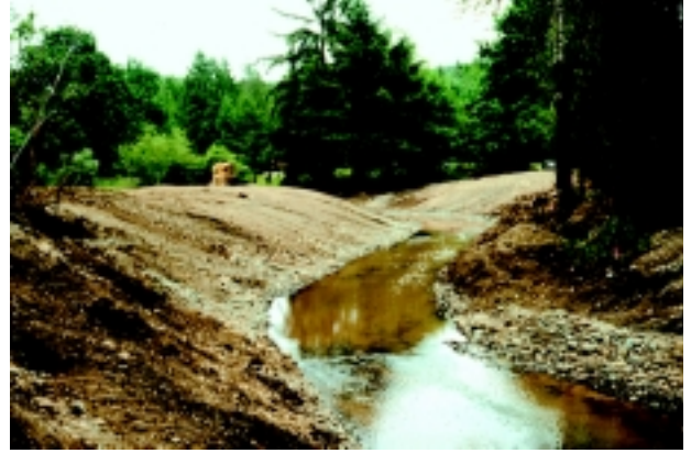
d. During construction, Creamer Slough, Tributary to Satsop River. 1998.
