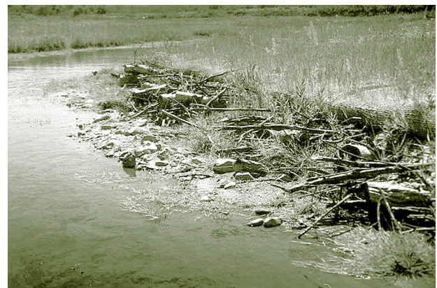
Figure 5-13. Gravel wrapped in biodegradable fabric serves as a deformable bank.
