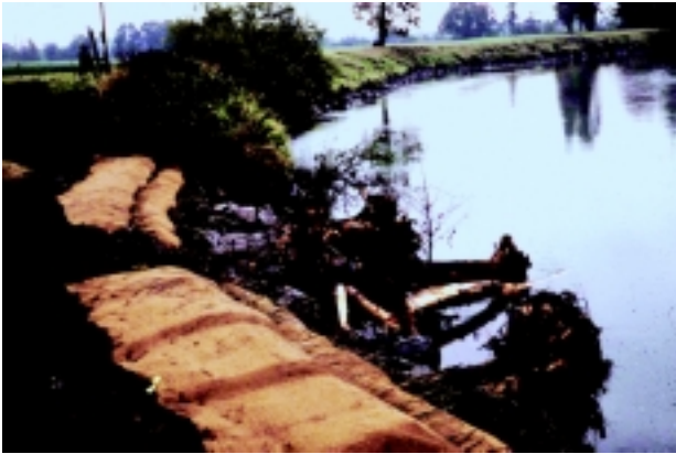
b. Roughened-Rock Toe with reinforced large woody debris, soil lifts and plantings. Nooksack River. 1999.
