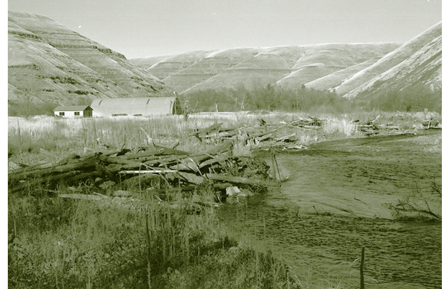
Figure 5-11. Engineered log jams on the Tucannon River.
