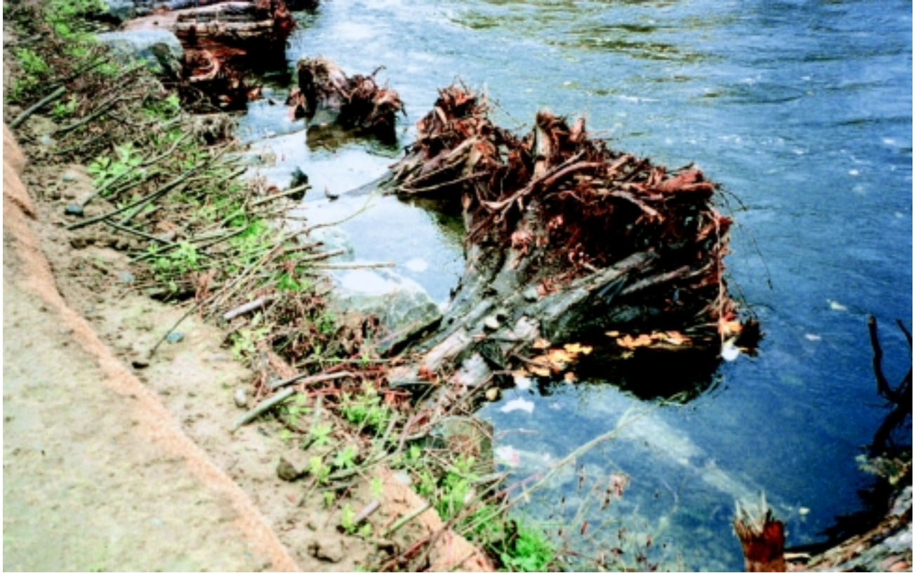
a. Log Toe with rootwads, boulders, soil reinforced lifts and plantings. One year after construction. Green River. 1994. Source: King County Department of Natural Resources.
