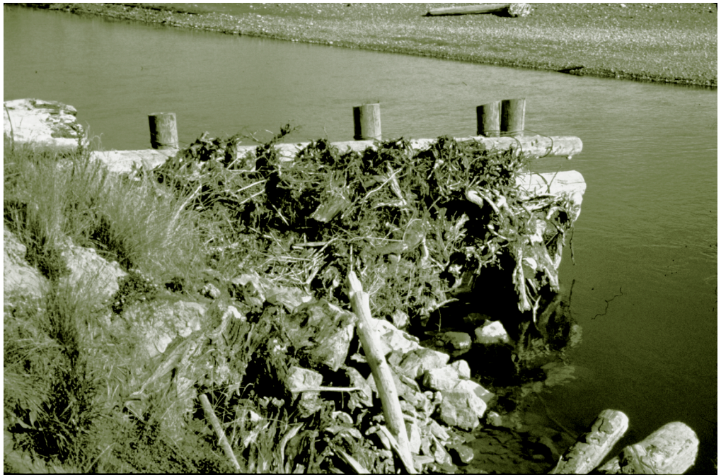
Figure L-4. Woody groins on the Nooksack River.
