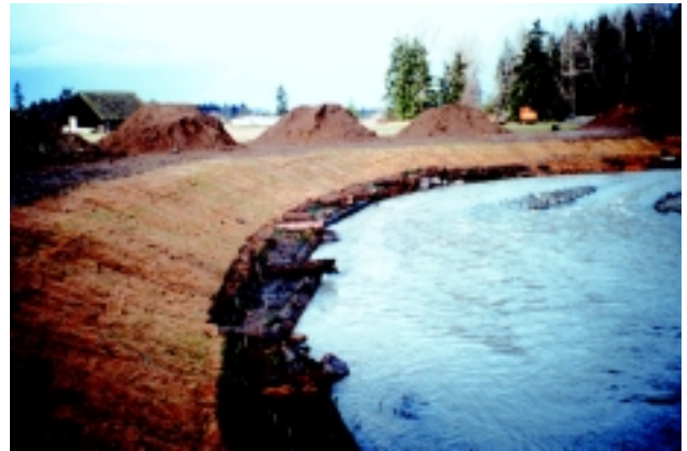
c. Log Toe with bank reshaping and plantings. Dungeness River. 1995.
