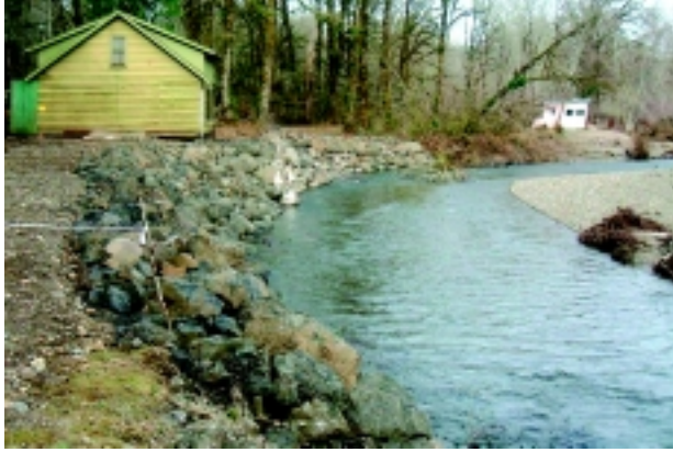
a. Riprap placed during an emergency. Tahuya River. 2002.
