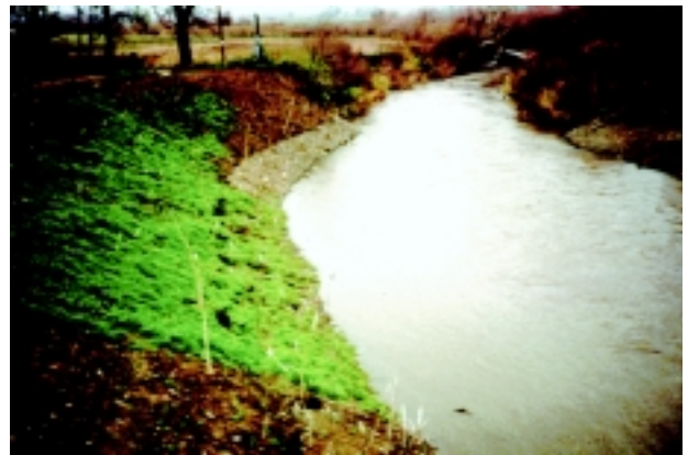
c. Bank Reshaping. Touchet River.
