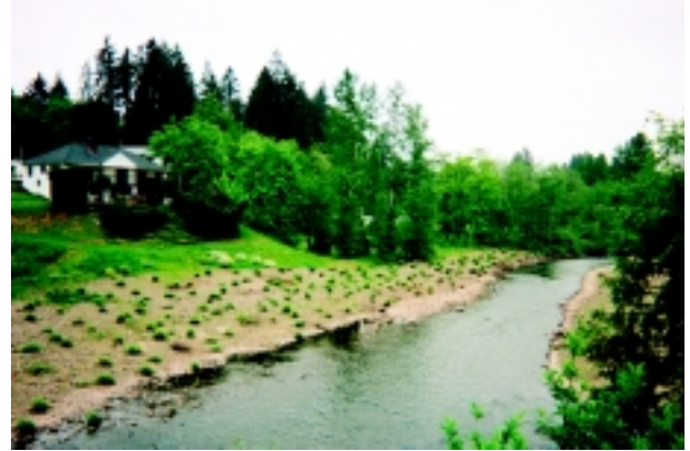
b. Floodplain Roughness. Woody plantings planted on floodplain for roughness. Salmon Creek, Tributary to Columbia River. Source: Inter-Fluve, Inc.
