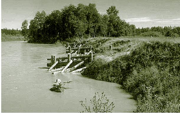
Figure 5-6. Log groins on the Nooksack River.
