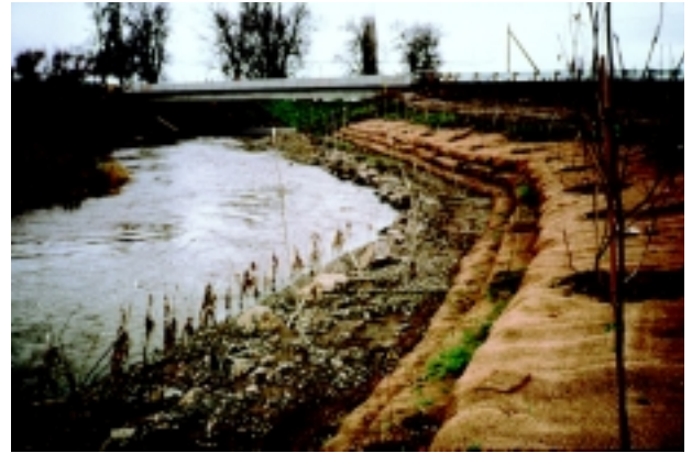
e. Roughened-Rock Toe with reinforced soil lifts and plantings. Touchet River. 2000.
