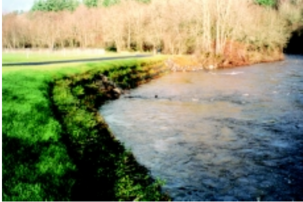
a. Soil Reinforcement lifts with barbs and rock toe. Salmon Creek, Tributary to Columbia River. 1997.
