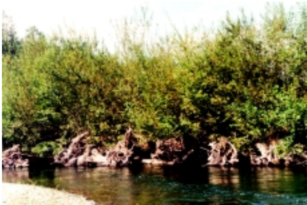
b. Log Toe with rootwads, boulders, soil-reinforced lifts and plantings. Four years after construction. Green River. 1998. Source: King County Department of Natural Resources.
