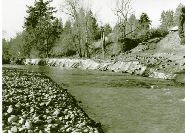
Figure 5-8. Eroding bank on Salmon Creek.
