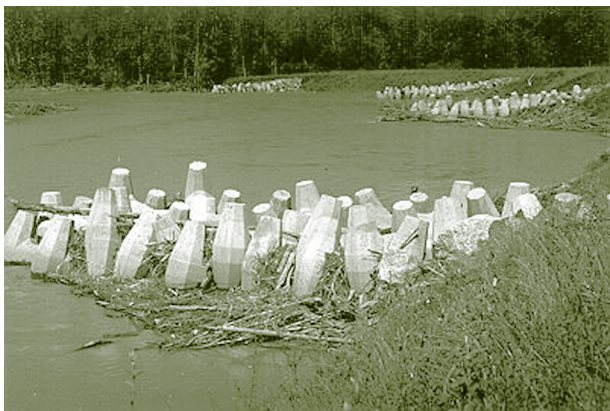
Figure 5-7. Concrete doloes with woody-material recruitment on the Nooksack River.
