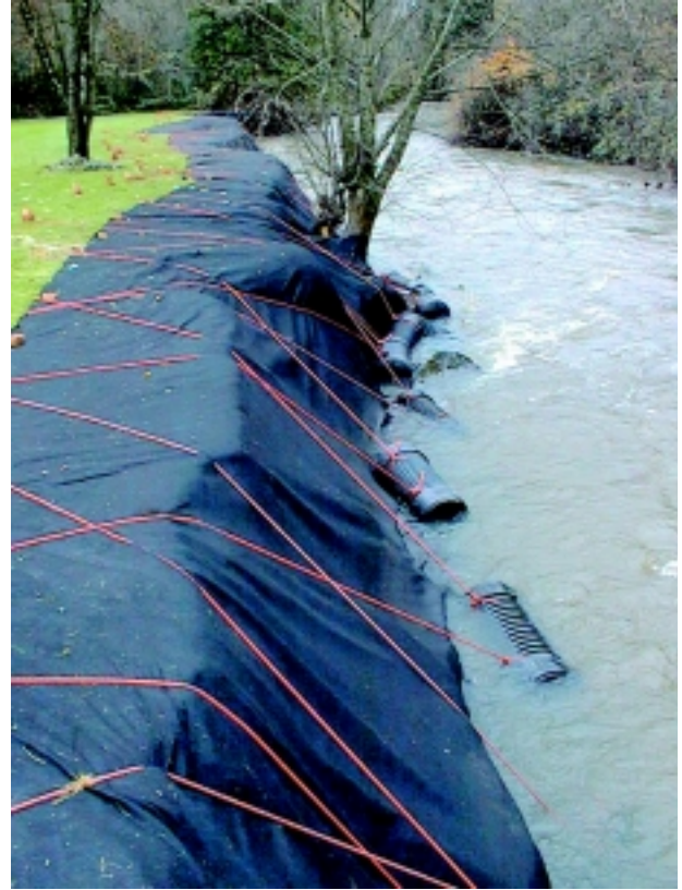
b. Temporary Manufactured Retention System using fabric mat. Salmon Creek, Tributary to the Columbia River. Source: Clark County Public Utilities.
