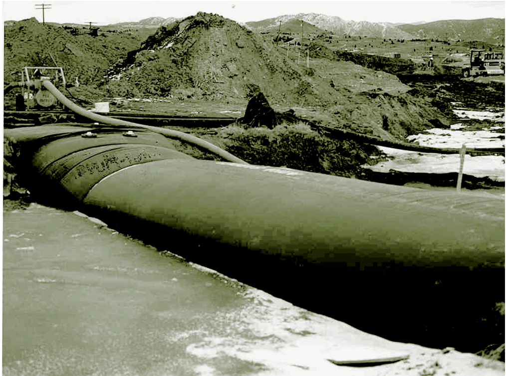
Figure M-1. An example of a water-filled geotube coffer dam in use.
