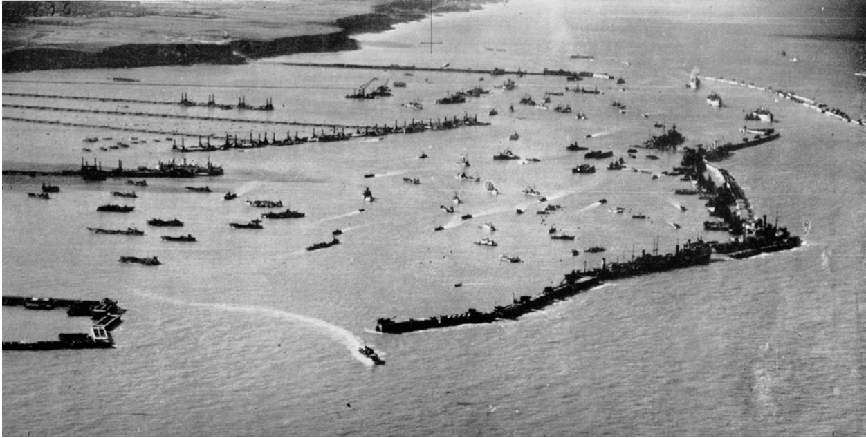
Figure I-3-14. Aerial photograph of the Mulberry "B" Harbor at Arromanches, France, June 1944 (from Institution of Civil Engineers, London, England, 1948, p. 242)
