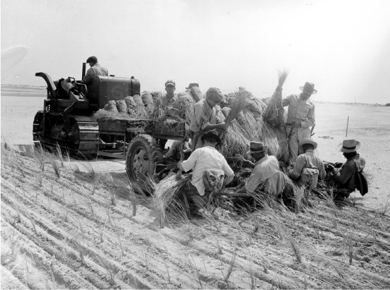
Figure I-3-12. Workers planting grass on a beach restoration project. The date and location of this image were not recorded, but the scene is likely the Outer Banks. Many dune and beach restoration efforts, sponsored by the National Park Service and other agencies during the late 1930s, also served as work relief efforts for a nation trying to recover from the Great Depression. Photograph from the Beach Erosion Board Archives
