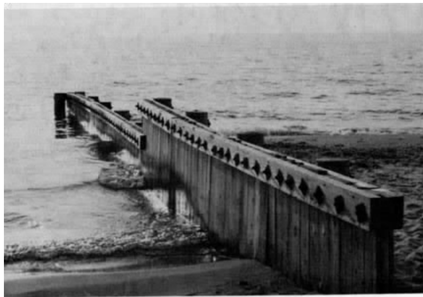
Figure 80 Timber Sheet Pile Groin
