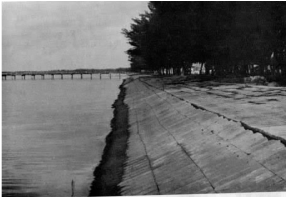
Figure 52 Lok-Gard Block Revetment
