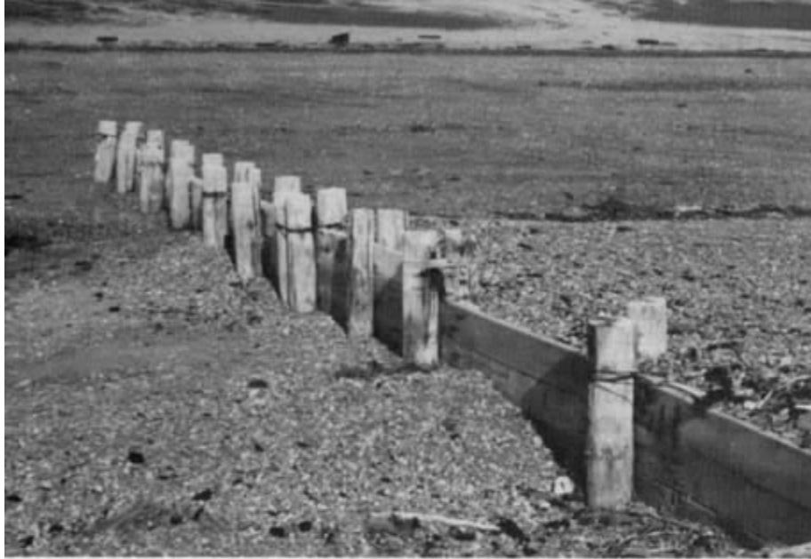
Figure 82 Timber Plank Groin
