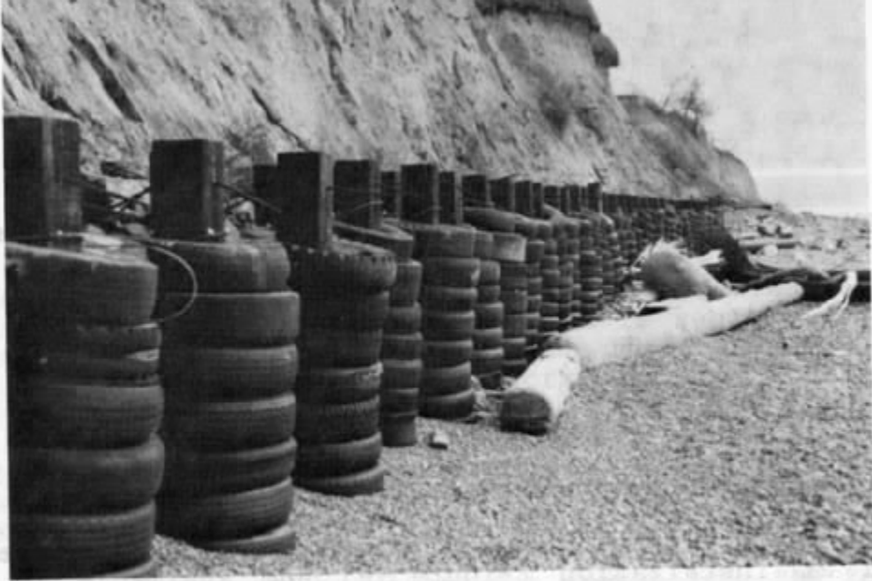
Figure 37 Used Rubber Tire and Post Bulkhead
