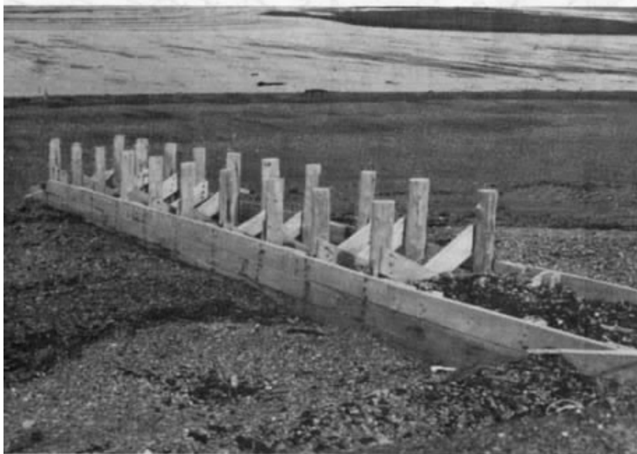
Figure 83 Timber Plank Groin
