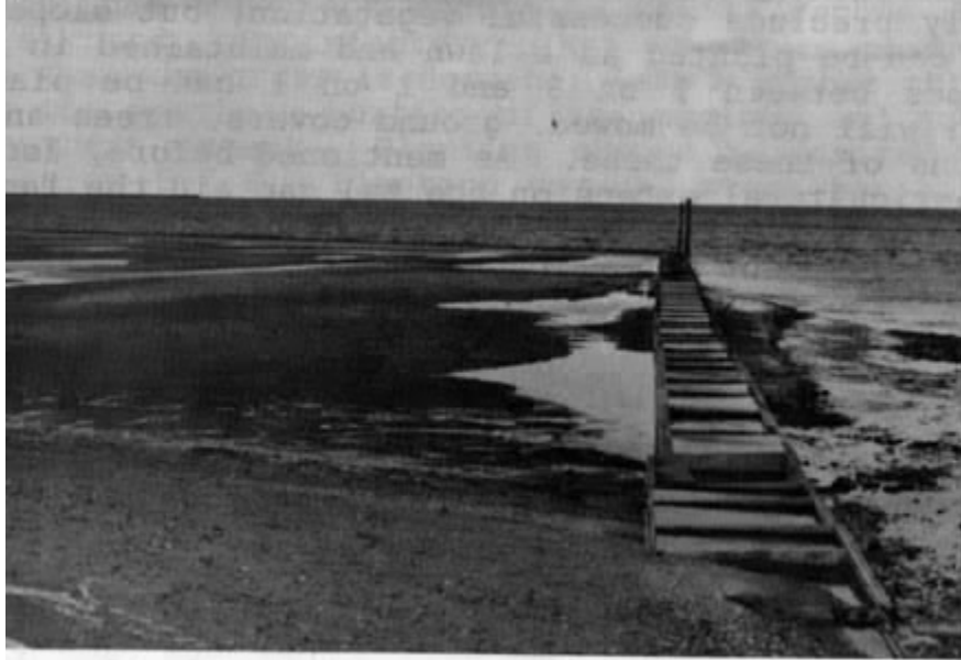
Figure 89 Concrete Box Sill
