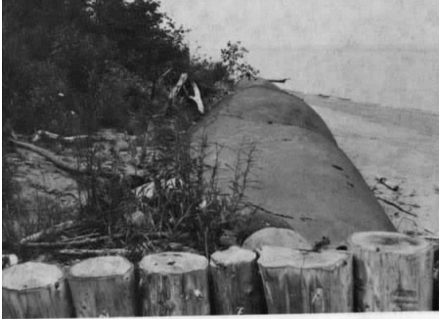
Figure 39 Longard Tube Bulkhead
