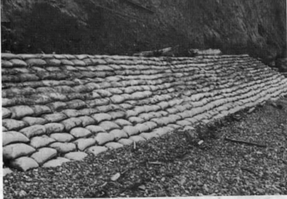
Figure 54 Stacked Bag Revetment
