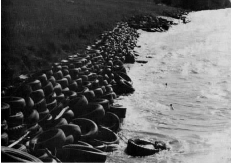
Figure 40 Stacked Used Tire Bulkhead
