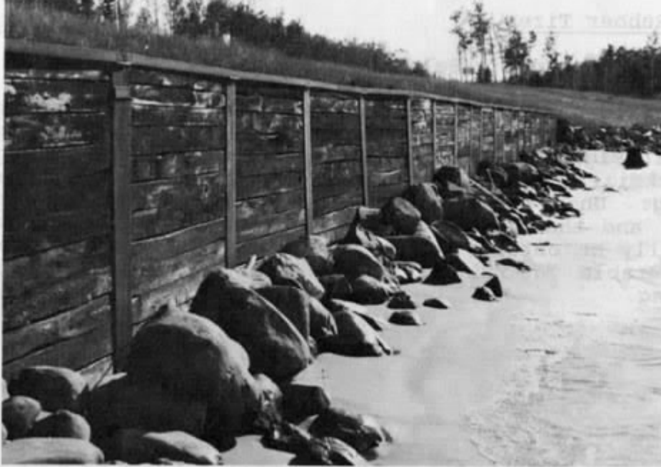
Figure 38 Railroad Ties and Steel H-Pile Bulkhead
