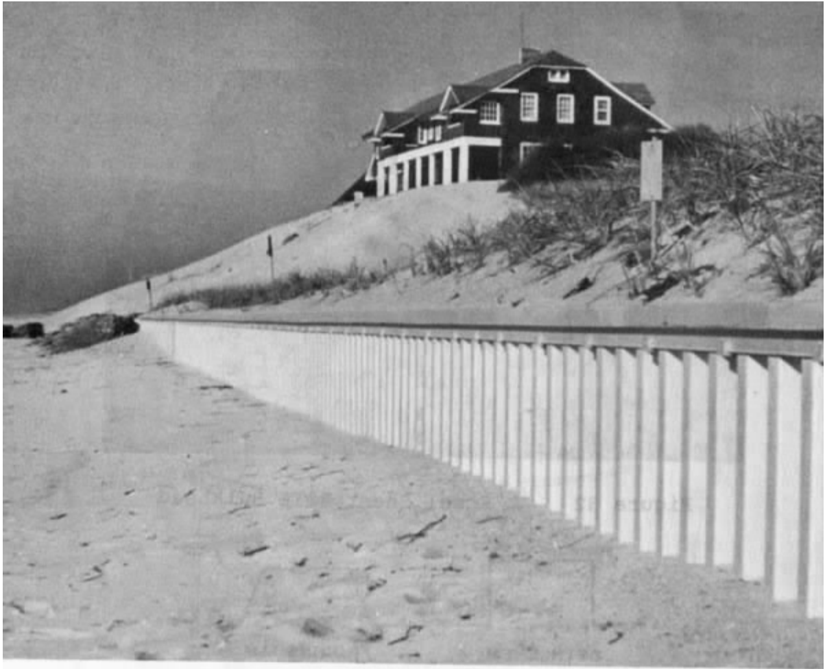
Figure 34 Aluminum Sheet Pile Bulkhead (Photo Courtesy of Koppers Company, Inc.)
