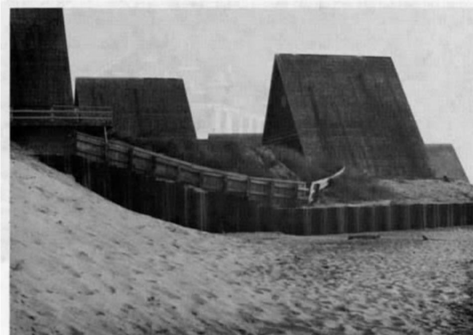
Figure 32 Steel Sheet Pile Bulkhead
