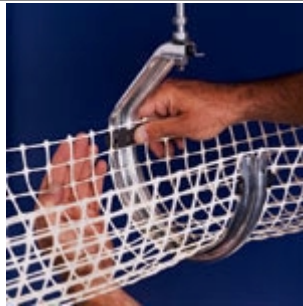
2. Plastic mesh in main support hanger and lock in with spring steel clip.
