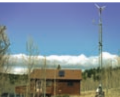
Location—A cabin in South Park, Colorado Capacity—600 watt Turbine manufacturer—Southwest WindPower Photo credit—E. McKenna, NREL/PIX04712
