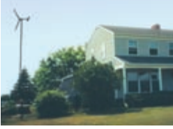
Location—A home in Charlotte, Vermont Capacity—10 kilowatts Turbine manufacturer—Bergey Windpower Company Photo credit—Trudy Forsyth, NREL/PIX09123
