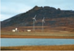
Location — Wales Wind Energy Project, Wales, Alaska Capacity — 0.1 MW Turbine manufacturer — Atlantic Orient Corporation Developer — Kotzebue Electric Association Photo credit — Steve Drouilhet, NREL/PIX09674
