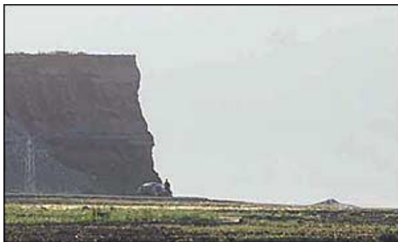
Failed Dam in Syria
