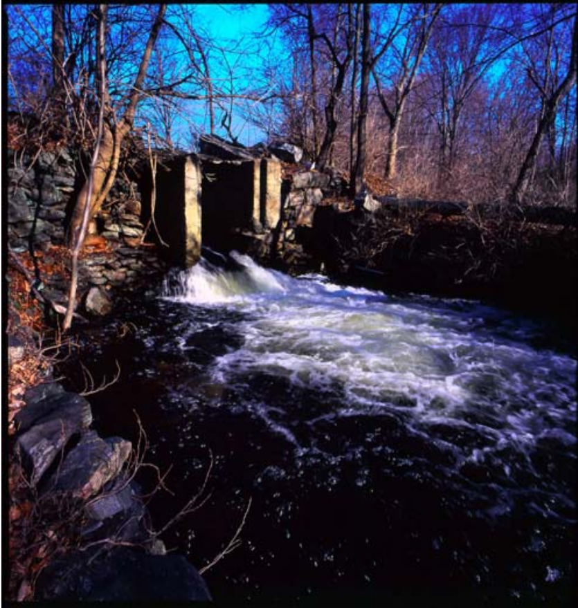
An old Colonial-era weir release spring flows from a pond in New England.
