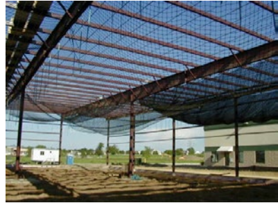
Safety nets used in construction sites.
