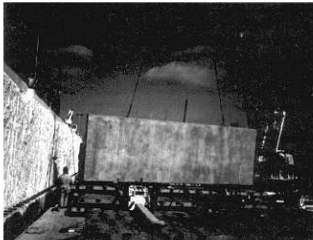
Figure 8-14. Installation of precast concrete stay-in-place forms at Lock 22, Mississippi River
