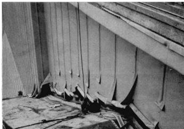
Figure 8-62. Installation of geocomposite, Pracana Dam
