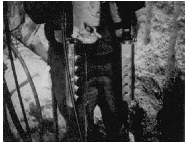
Figure 5-13. Piston-jack splitter
