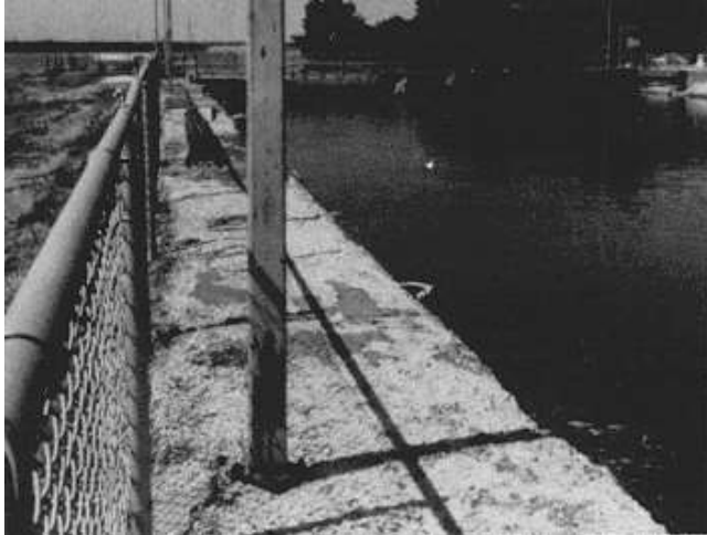
Figure 2-18. Severe scaling
