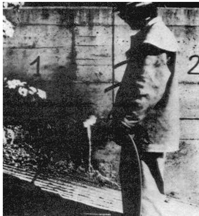
Figure 5-6. Thermal lance
