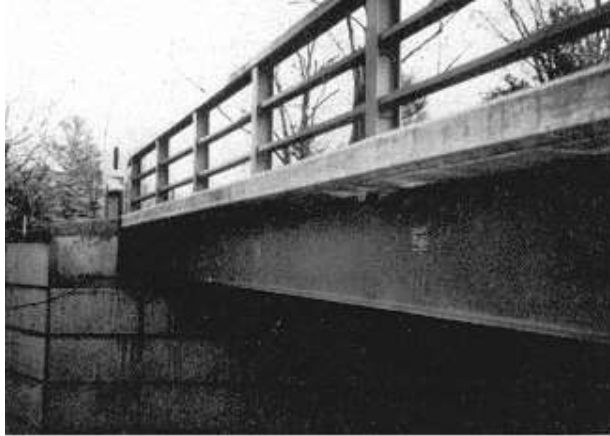
Figure 8-53. Precast abutment and deck units, Ulsterville Bridge
