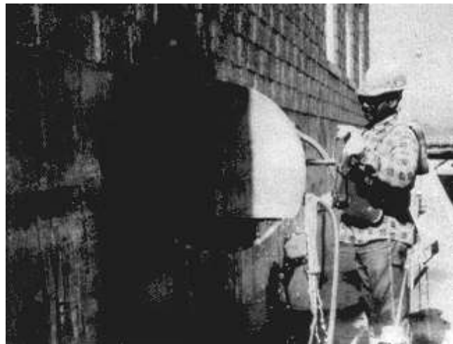
Figure 5-3. Diamond-blade saw
