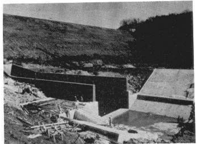
b. After repair
