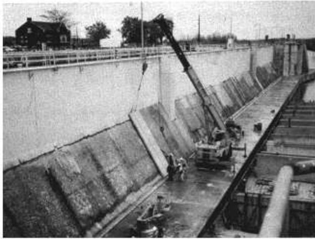
a. Installation of precast concrete panels
