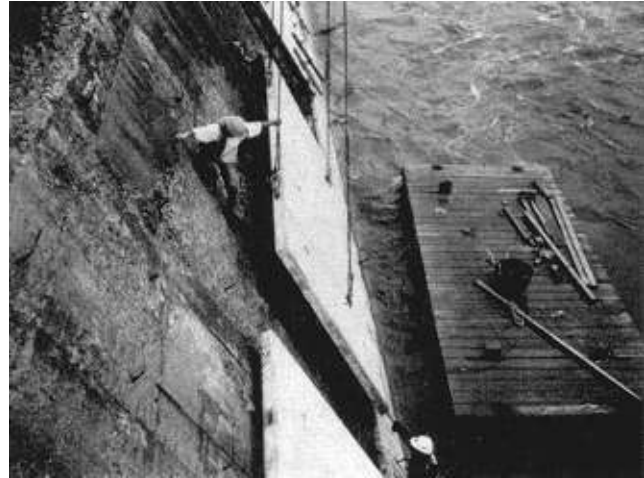
Figure 8-17. Installing precast concrete panels used to overlay the back side of the river wall at Troy Lock, Hudson River (Miles 1993)
