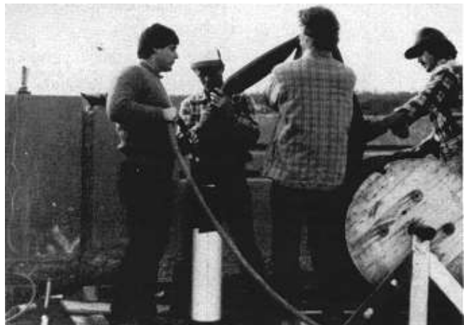
Figure 8-23. Two-component natural rubber and elastomer coated nylon sleeve being inserted into drill hole, Bagnell Dam
