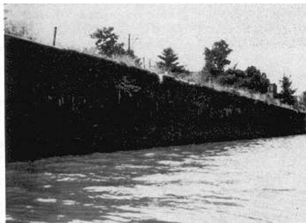
a. Overall view
