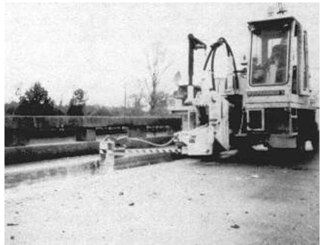
Figure 5-8. Spring-action hammer (mechanical sledgehammer)
