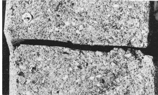
Figure 2-23. Loss of joint sealant
