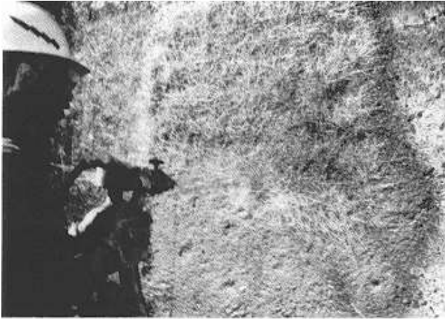
a. Applying the coating with equipment that simultaneously sprays the mortar from one nozzle while it chops and blows the fiber from a cutterhead
