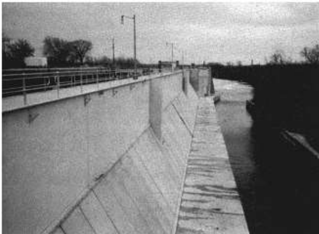
b. River wall complete with precast concrete panels
