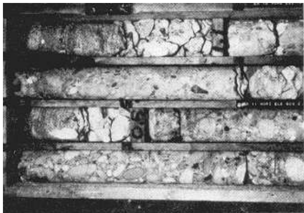
a. Portions of the core from two drill holes through river chamber wall which had been refaced with shotcrete
