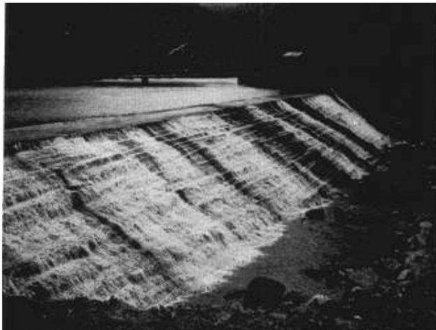
Figure 8-64. Condition of RCC following periodic overtopping, Ocoee No.2 Dam
