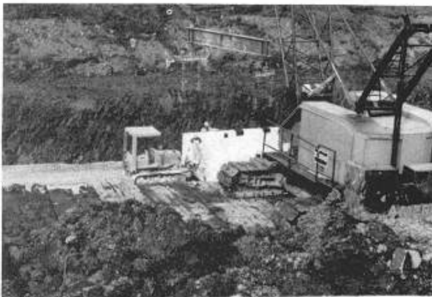
Figure 8-47. Channel section delivery and installation, Blue River Channel
