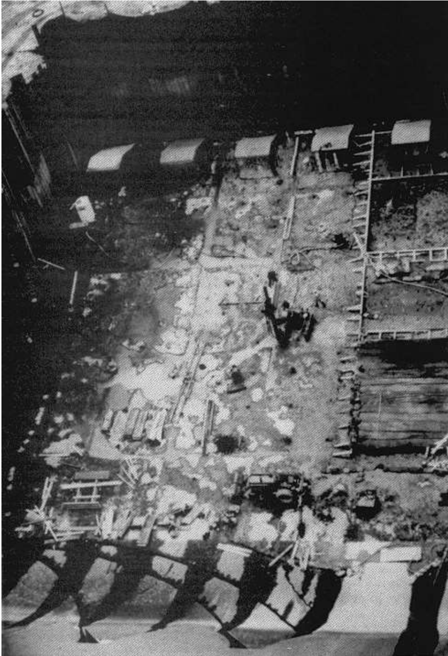
Figure 8-34. General view of repair operations, Kinzua Dam, 1974
