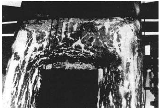
Figure 2-24. Efflorescence
