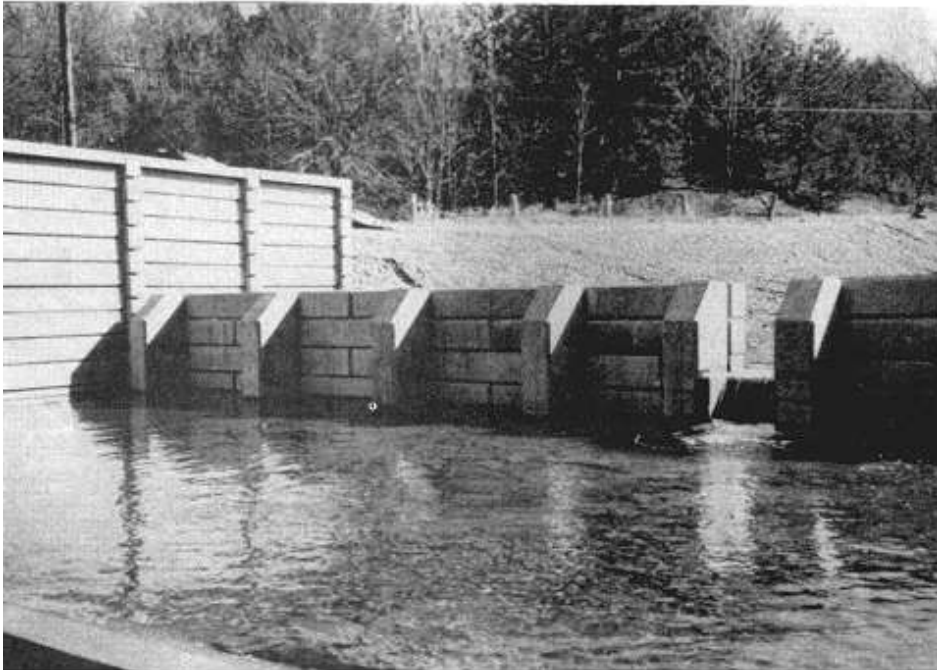
Figure 8-43. Precast concrete checkdams, Chauncy Run
