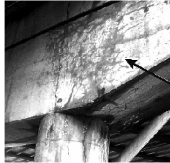
DEF Cracking
