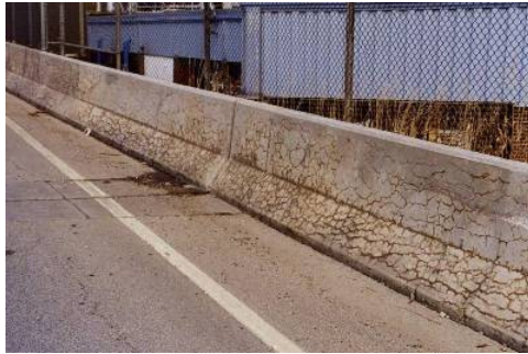
ASR Cracking
