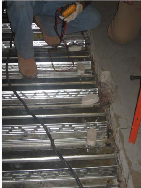
Vector Corrosion Galvashield "Puck" Installation
