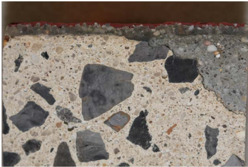
Painted Epoxy Topping
