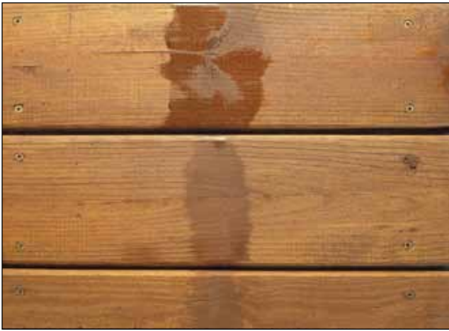
Figure 16–20. Lap marks on wood finished with semi-transparent stain.
