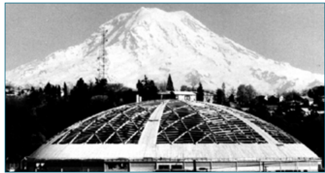
Figure 17-8. This 161.5-m- (530-ft-) diameter Tacoma dome (Tacoma, Washington), built in 1982–1983, is one of the longest clear roof spans in the world. (Photo courtesy of Western Wood Structures, Inc., Tualatin, Oregon.)
