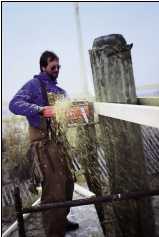
Figure 13-2 Typical pile notching process. Photograph by Patty McDaniel.
