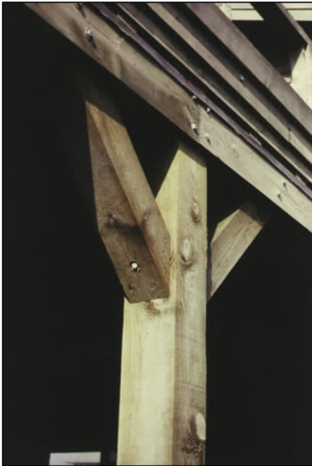
Figure 13-9 Knee bracing in a wood-pile foundation.
