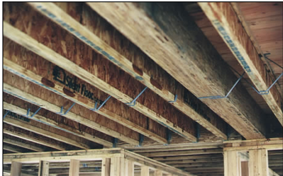
Figure 13-24 Plywood web I-beams used as floor joists with metal brace used to keep the bottoms of the joists from twisting. Also note glue-laminated beam.
