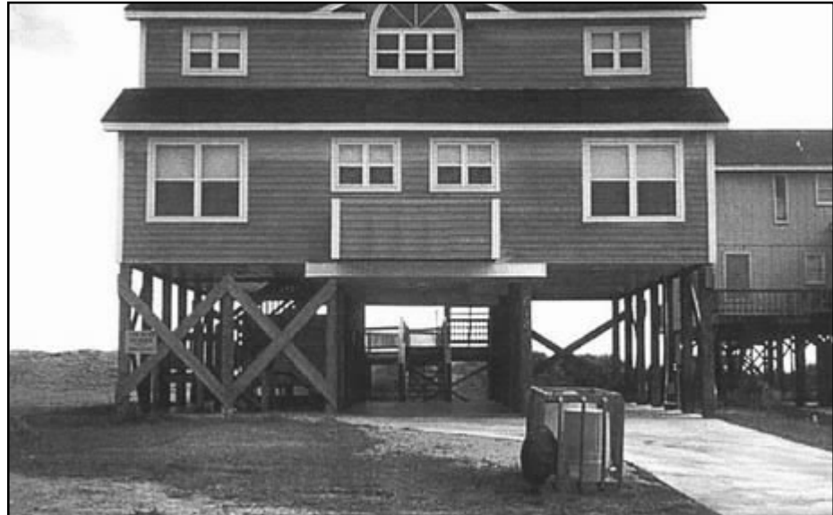
Figure 13-8 Diagonal wood bracing in a wood-pile foundation.
