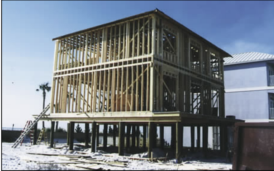
Figure 13-7 Typical wood-pile foundation.
