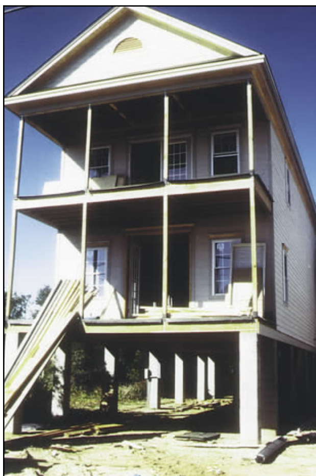
Figure 13-10 Open masonry foundation.
