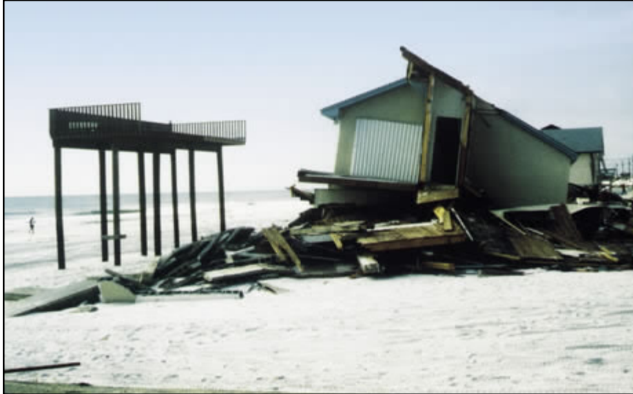
Figure 13-29 Building damage from Hurricane Opal at Pensacola Beach, Florida. The deck, which was constructed to State of Florida Coastal Construction Control Line (CCCL) design requirements, survived; the building, which was not constructed to CCCL requirements, did not survive. See Appendix G for a discussion of the Florida CCCL.
