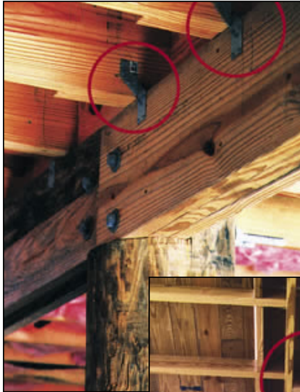
Figure 12-52 Wood joist/beam connector.
