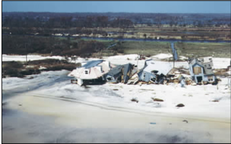
Figure 12-14 Hurricane Fran (1996), North Carolina. Building collapse caused by the force of water flowing through an inlet created across Topsail Island during the storm.
