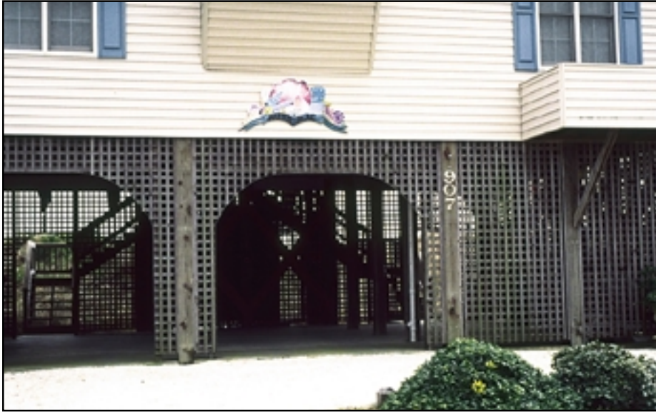
Figure 12-73 Lattice installed beneath an elevated house in a V zone.
