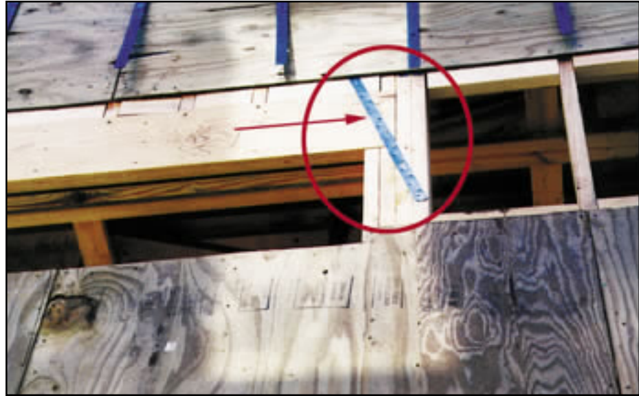
Figure 12-42 Metal connector at window opening.
