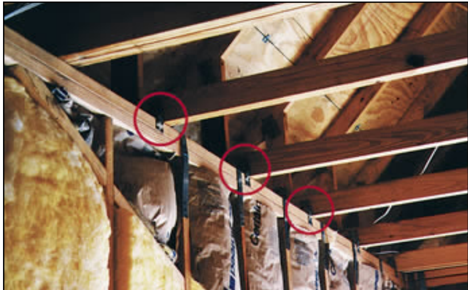
Figure 12-35 Typical connection of truss to wood wall.
