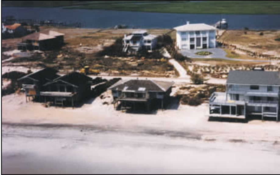
Figure 12-13 Hurricane Fran (1996), North Carolina. Building that moved off its foundation. Original location indicated by black line. Note that the porch roof failed on the house on the left.
