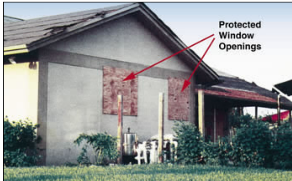
Figure 12-6 Hurricane Andrew (1992), Dade County, Florida. Openings in house protected with plywood panels.
