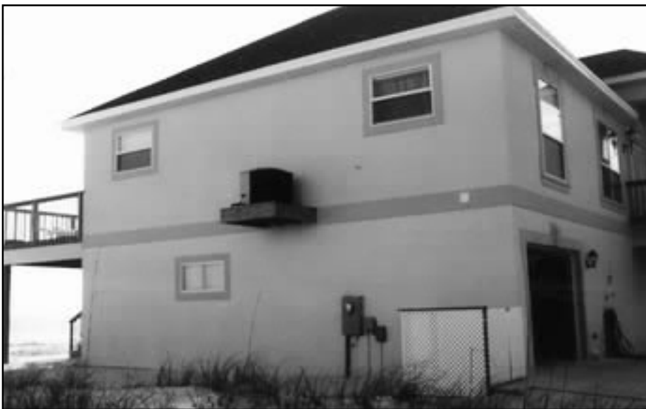
Figure 12-115 Proper elevation of mechanical equipment in a flood-prone area.
