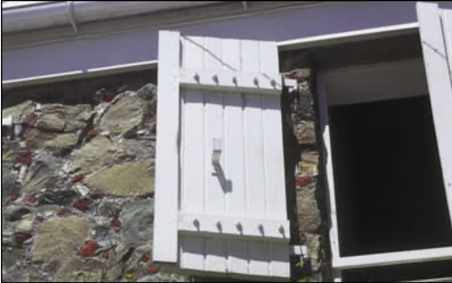
Figure 12-98 Hurricane Marilyn (1995), U.S. Virgin Islands. Shutters constructed of 2x4 lumber.
