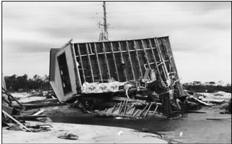
Figure 12-8 Hurricane Fran (1996), North Carolina. House overturned by flood and wind forces.
