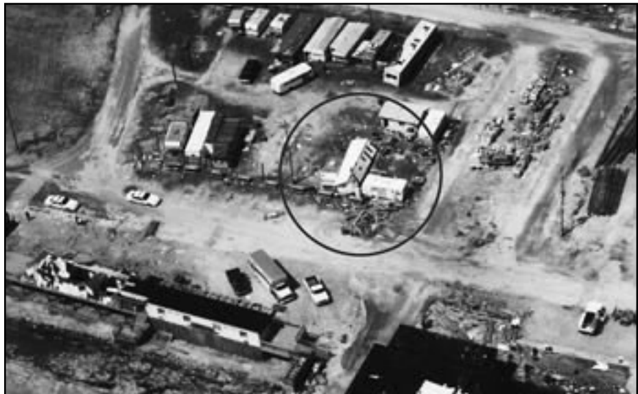
Figure 12-9 Hurricane Fran (1996), North Carolina. Lightweight building (manufactured home) overturned by wind forces.
