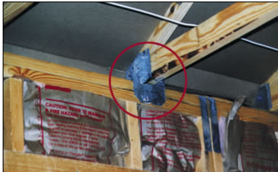
Figure 12-36 Typical connection of truss to wood wall.
