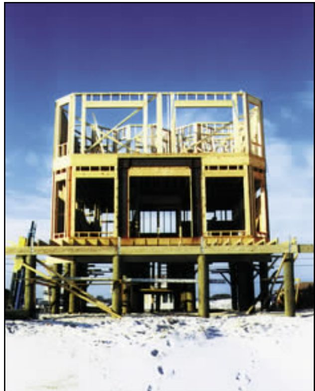
Figure 12-49 Steel moment frame at large opening.
