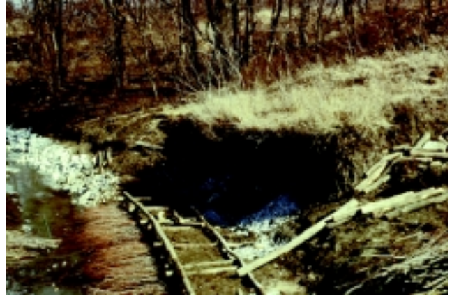
Figure 16-15b A live cribwall during installation
