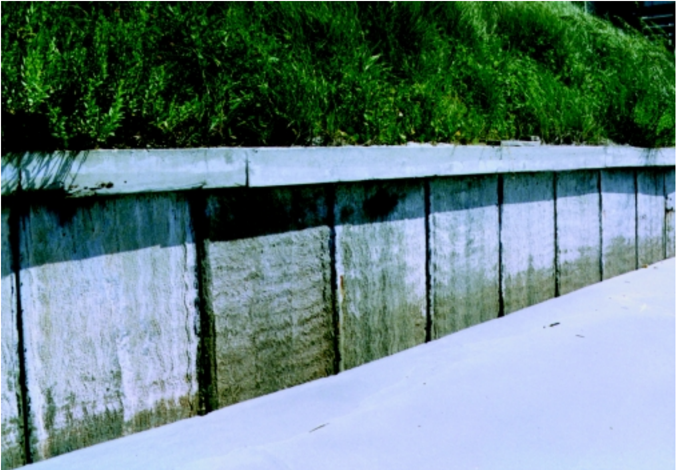
Figure 16-49 Concrete bulkhead system
