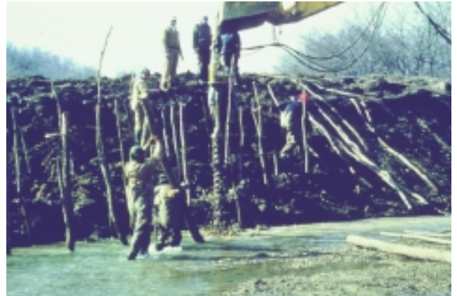
Figure 16-25b Installing dormant posts (Don Roseboom photo)
