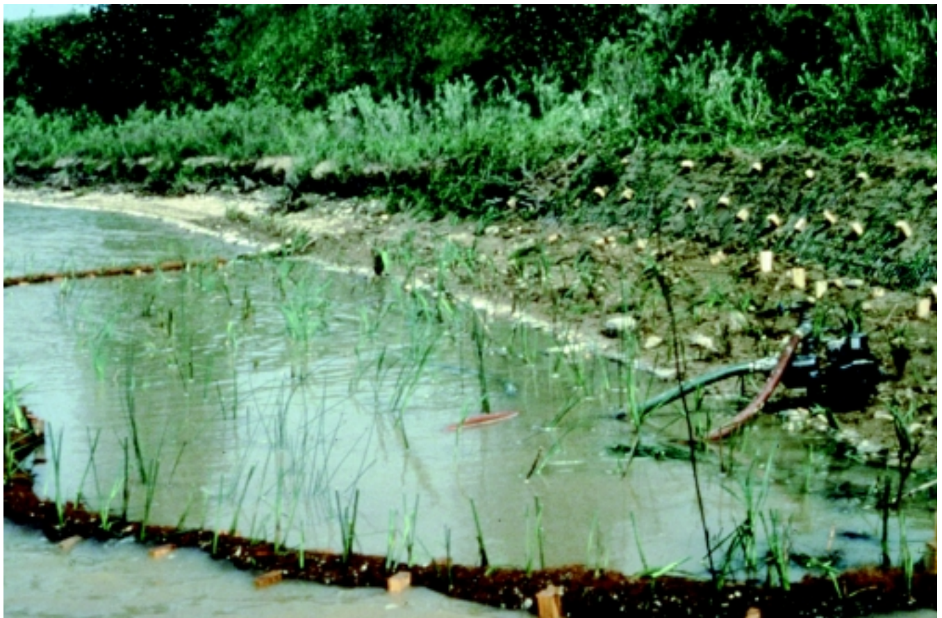
Figure 16–57 Coconut fiber roll system
