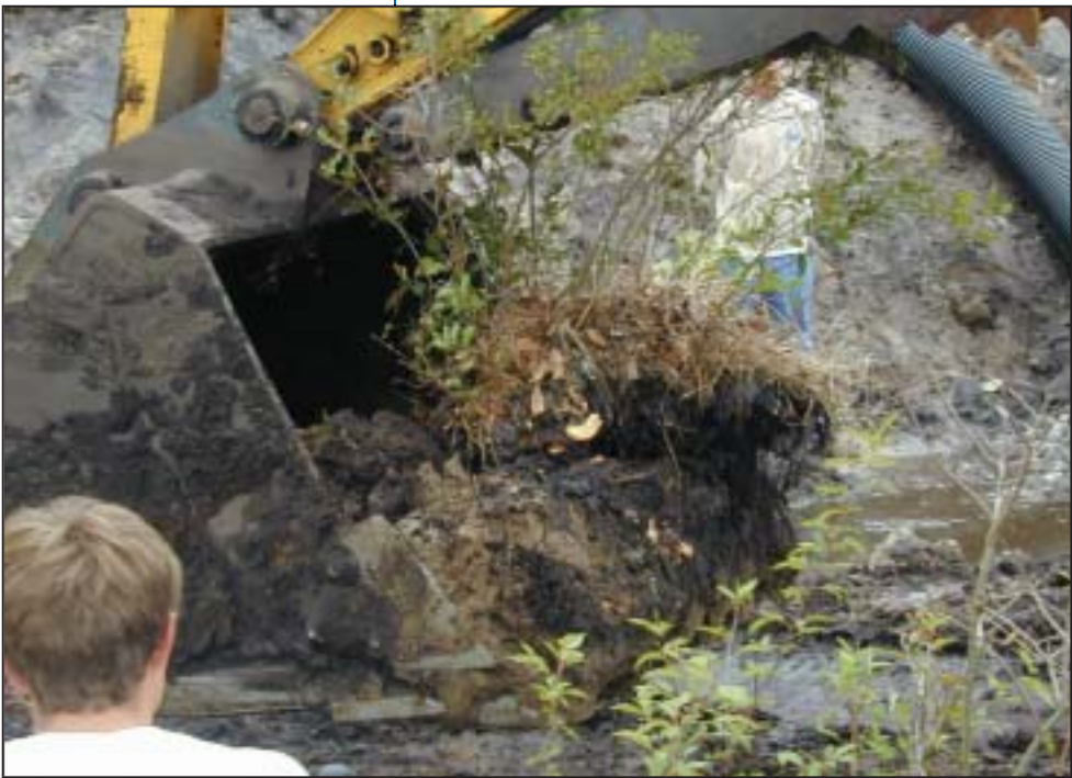
Figure 9.1 Salvaging vegetation at construction site
