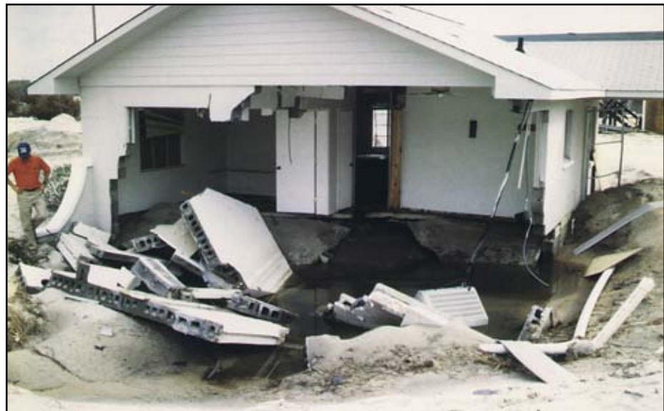
Figure 7-52 Hurricane Fran (1996). Extreme case of localized scour undermining a slab- on-grade house on Topsail Island, North Carolina. The lot was several hundred feet from the shoreline and mapped as an A zone on the FIRM prior to the storm. This case provides one argument for the treatment of these areas as coastal A zones.
