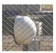
Microwave intrusion detectors – Highly sophisticated transmitters and receivers used to detect the motion of people between the outer and inner protected area fences. A microwave
