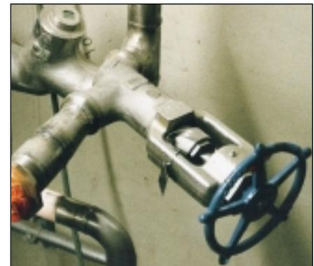
Class 2500 hermetically-sealed Y-pattern bellows sealed valves.
