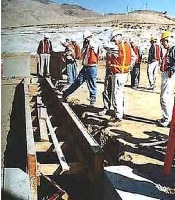
Figure 9: Senior members of an Expert Board of Consultants inspect the construction of a cut-off wall in the foundation of a large dam for conformance with design specifications.
