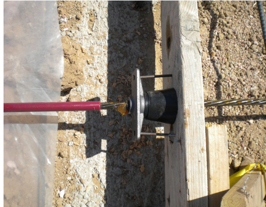
Source: JWK Inspections
