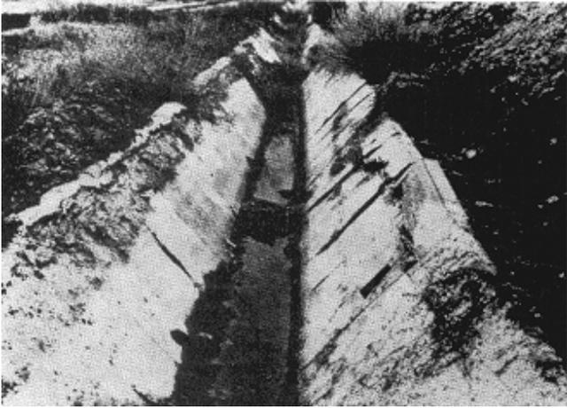
**Figure 2-14. Disintegration of concrete caused by sulfate attack**
