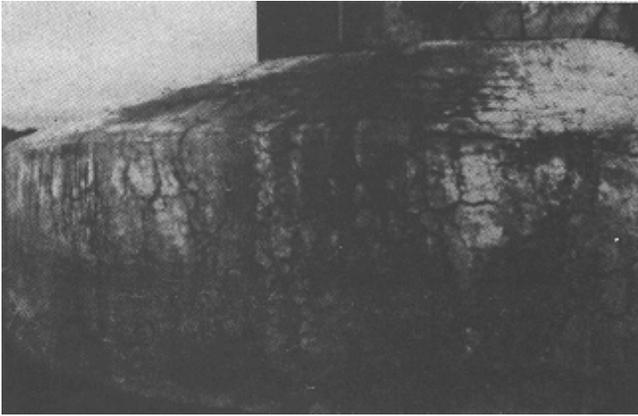
Figure 2-7. Pattern cracking caused by alkali-carbonate reaction
