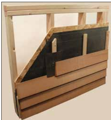
Figure 16-15. Demonstration of siding installation over a secondary drainage plane (rain screen) showing wall studs, sheathing, water-resistant barrier (WRB), furring strips, and interleaved WRB at the butt joint. Note that the butt joint is centered directly over the furring strip and the underlying stud and the end grain has been sealed.
